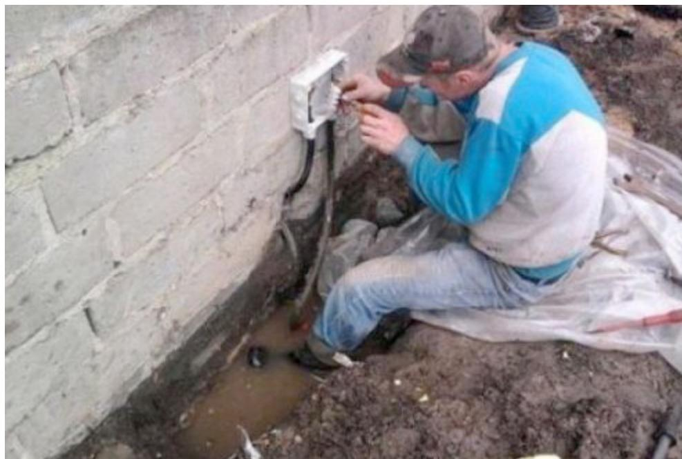
You don't have to be an electrical engineer to recognize that it's not a great idea to repair electrical equipment with one's feet immersed in a puddle. It's just too bad the gentleman in the photo didn't get the memo.
