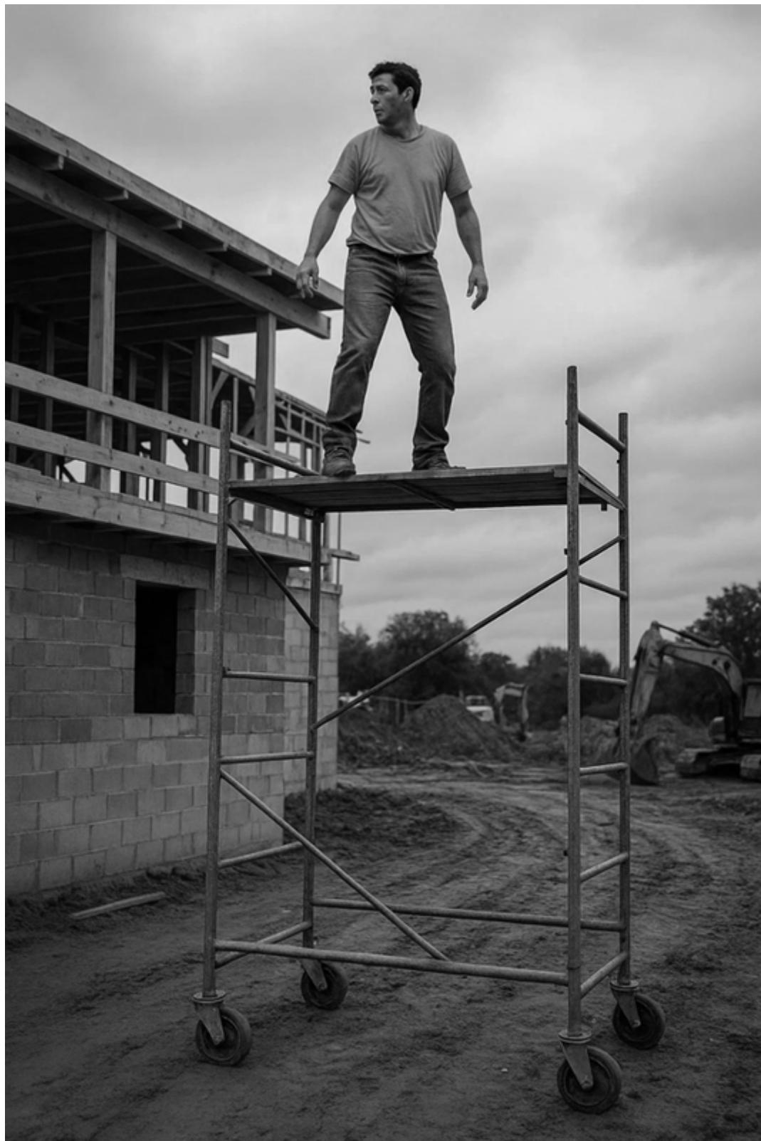
This image highlights a major scaffold tower safety issue. The individual is standing on a scaffold platform without any guardrails, fall protection, or visible stabilization.
