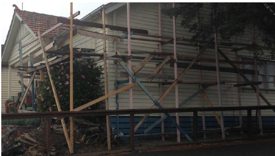
Here's another 'pirate's plank' at a construction site. It appears that while workers can see the windows, they can't always see the light when it comes to ensuring their own safety. One small misstep could have disastrous consequences. Where's the proper scaffolding that is required by law? (WorkSafeVictoria, Australia)
