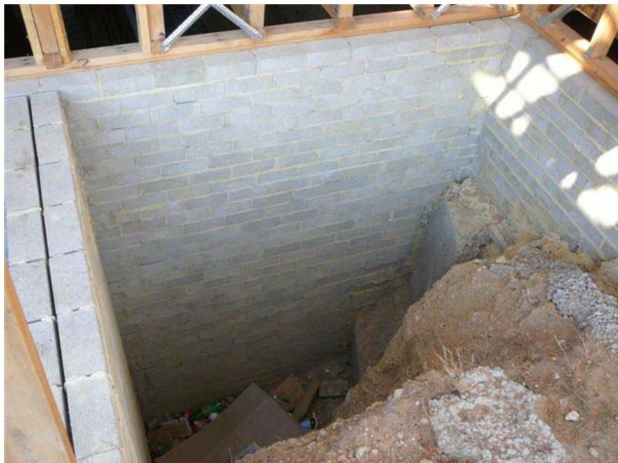
Here we have an open, unprotected hole in the ground, complete with bricks that could make the ride down even more “interesting.” This situation could easily result in a serious injury or fatality, but it’s easily preventable by building a guard around this hazard. (WorkSafeVictoria, Australia)
