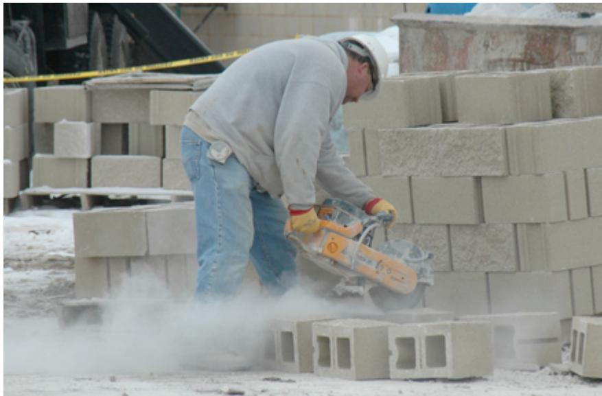
Head protection: check. Hand protection: check. Two out of three ain't bad, as the saying goes, but in this case the critical missing PPE element is respiratory protection. This worker is kicking up a lot of dust as he uses a concrete saw. We wouldn't want to be on the breathing end of this arrangement. Ongoing exposure to silica dust can lead to deadly silicosis and lung cancer. Use of appropriate respiratory PPE is essential in preventing silica exposure.
