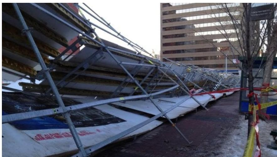
Wind gusts exceeding 120 kilometers (75 miles) per hour sent scaffolding crashing down at a construction site in Edmonton, AB. Fortunately, no workers or members of the public were injured. High winds can make conditions hazardous for construction workers, and in the case of building materials being thrown, can also endanger the public. (CBC News)
