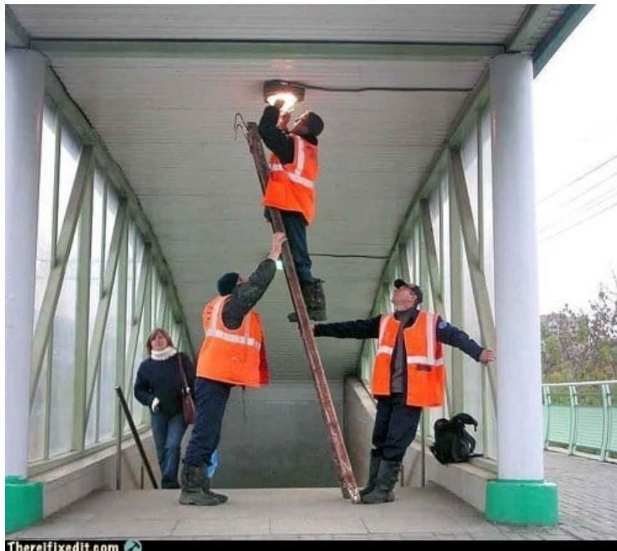
This photograph may bring to mind a joke along the lines of "How many workers does it take to screw in a light bulb?" but from a safety standpoint, there's not much that's funny about it. A sideways slip of the ladder, especially in the direction of the stairwell, could have fatal results for the worker on the ladder and anyone walking on the stairs. A real stepladder is what's needed here. (Photo re-used with permission from Cheezburger.com)
