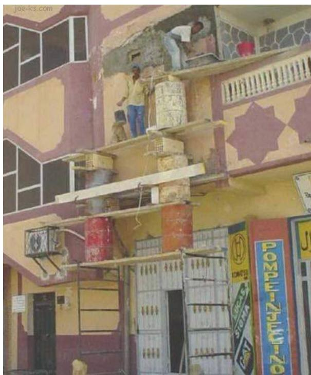
Scaffold safety has plunged to a new low in this photo. Barrels and boards stacked high have created a precarious working platform for these two workers. Like a house of cards, everything could come crashing down at any moment. (Source unknown)
