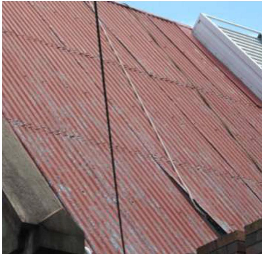
A safety inspector visited a church roofing project after receiving a complaint about unsafe conditions and quickly shut down the project after observing safety rope running over the sharp surfaces of the metal roof edge. It would have only been a matter of time before the sharp edge severed the rope, with potentially deadly consequences. (WorkSafeVictoria, Australia)
