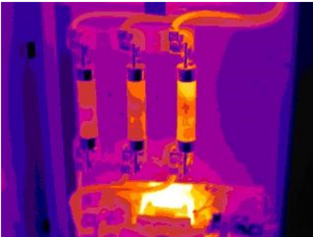
Iron palette of fuse bus bar
