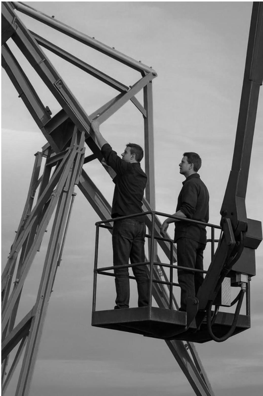
This image shows two workers on a mobile elevated work platform (MEWP), but several safety concerns are visible. Neither worker is wearing a safety harness or fall arrest system, which is essential
