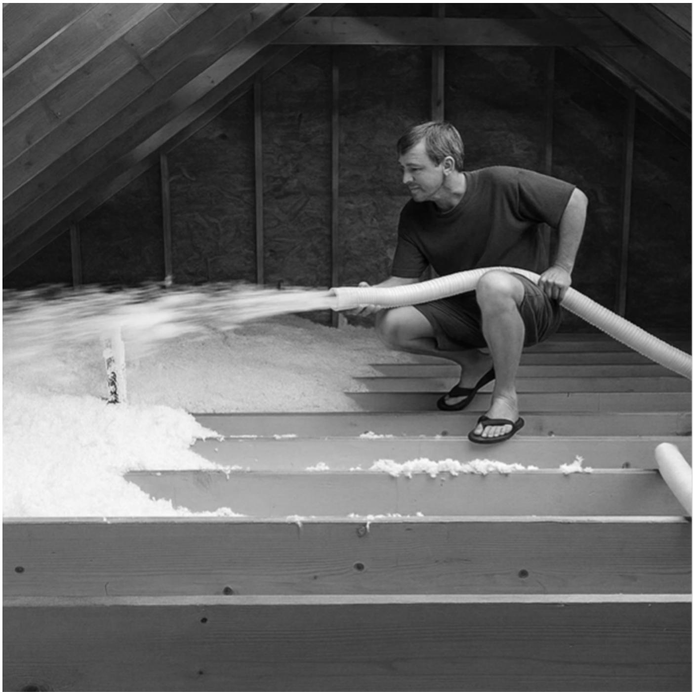
The worker is applying insulation in an attic without any visible personal protective equipment (PPE). He is wearing a t-shirt, shorts, and flip-flops, leaving his skin completely exposed. There's also no sign of a dust mask, goggles, or gloves—all essential when working with loose-fill insulation, which can
