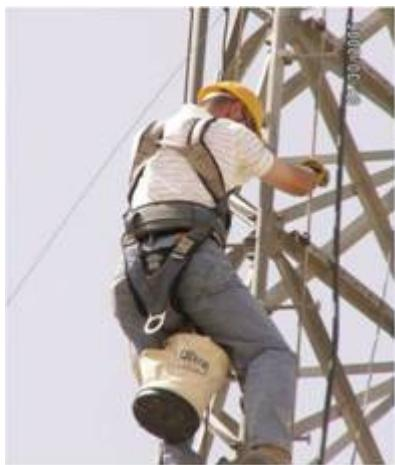
The good news: The worker scaling this elevated structure is using personal fall arrest equipment. The bad news: His body harness is *upside down*—the D ring should be positioned at the center of his upper back, not below his behind!
