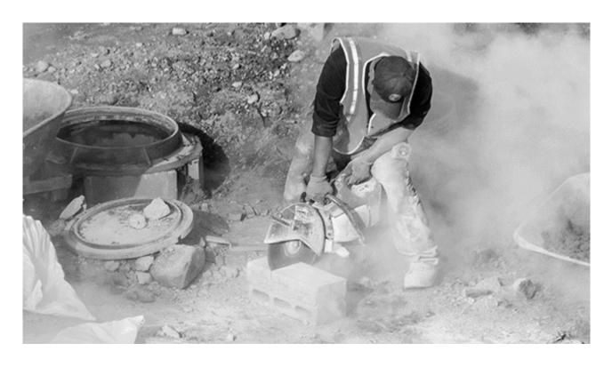
What's wrong in this picture? There is a construction worker who is working around excessive dust and he is not wearing any proper PPE to avoid dust hazards.
