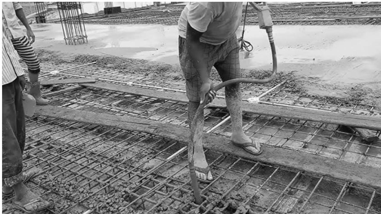
Concrete work may seem routine, but it comes with serious hazards if safety practices are ignored. In the image, the worker is using a concrete vibrator while wearing flip-flops and standing directly in wet concrete—this exposes them to both chemical and physical risks. Wet concrete is highly alkaline and can cause severe skin burns or dermatitis with prolonged contact.
