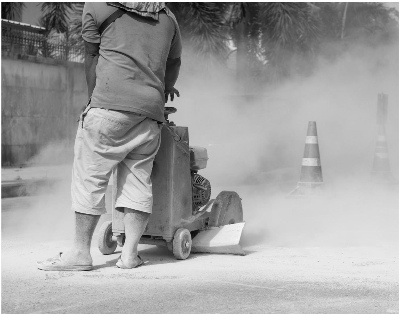
In the image, a worker is operating a concrete cutting machine in a cloud of dust without any visible personal protective equipment (PPE). The worker is exposed to respirable crystalline silica, which can cause serious lung diseases like silicosis. Additionally, the person is wearing open-back shoes and no gloves, leaving feet and hands vulnerable to sharp debris or contact with the machine.
